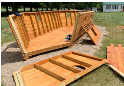
Building progression of new ark play structure built and dedicated in the Wilderness area
